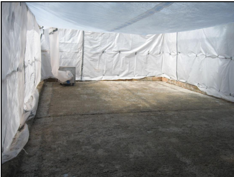
Completed conductive flooring removal at BLA Building 412. March 2011.
