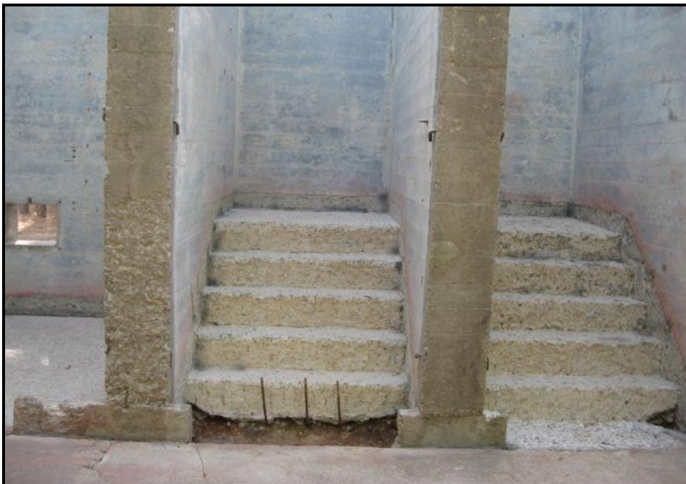
View of above (Building 8102-4) following conductive flooring removal. February 2011.
