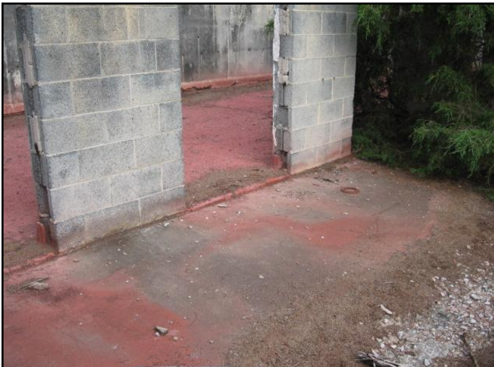
View of conductive flooring stains on sidewalk at BLA Building 405. October 2009.
