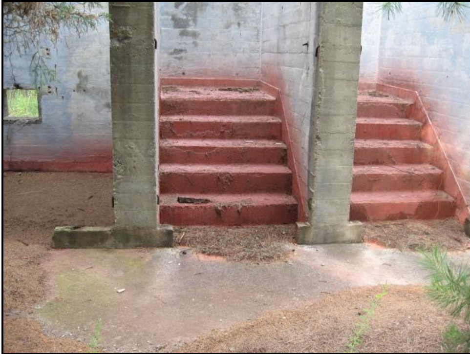
Conductive flooring inside Building 8102-4. August 2008.
