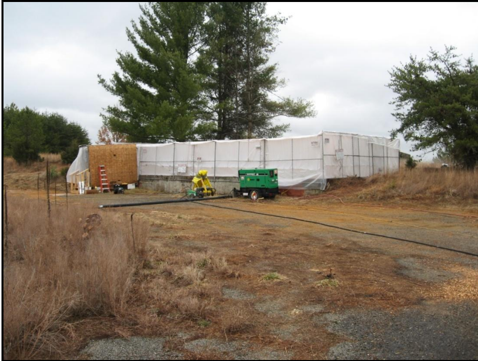
Asbestos containment unit set up at BLA Building 412. March 2011.
