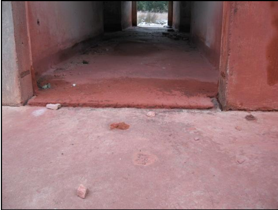
View of conductive flooring material inside BLA Building 404. October 2009
