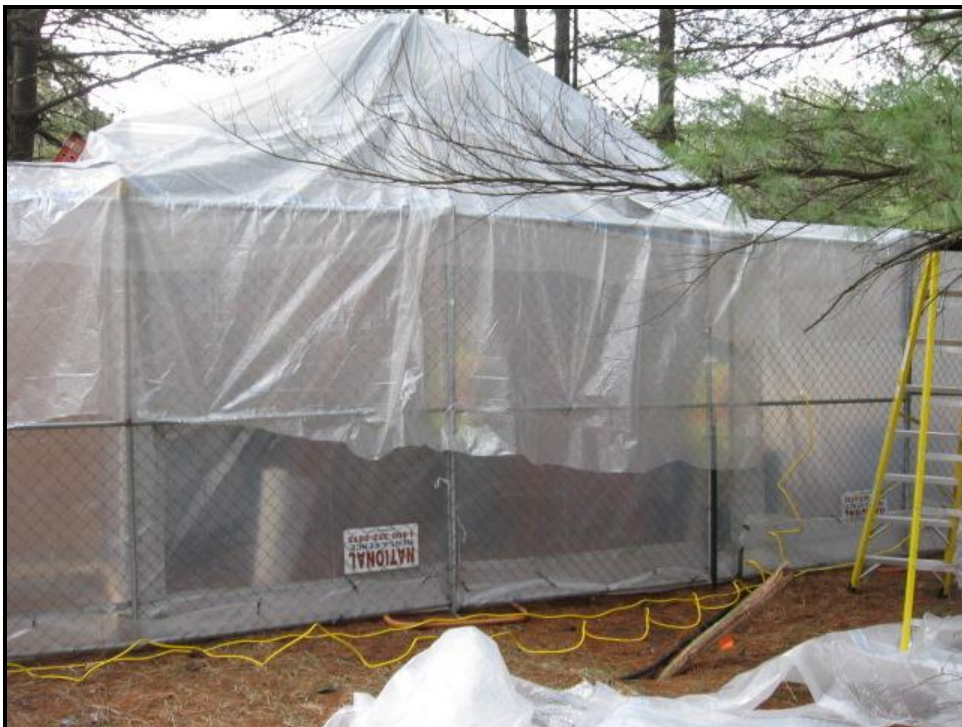
Winter Environmental crew erecting asbestos abatement enclosure at Building 1. January 2011.
