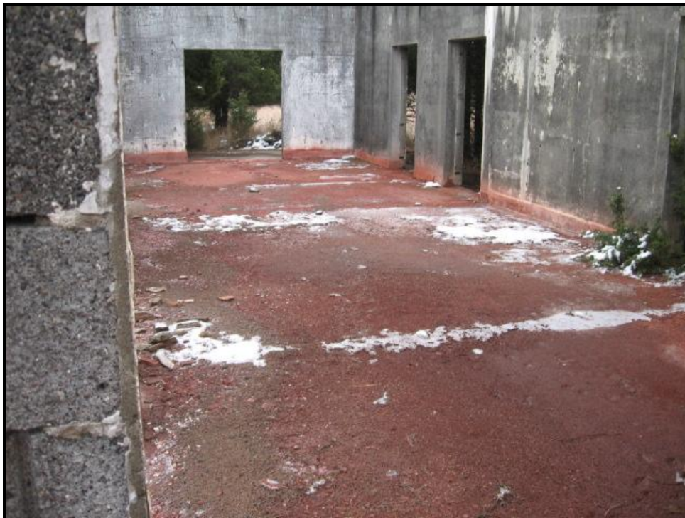
View of conductive flooring inside Building 404. January 2011.
